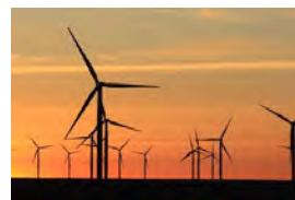
Figure 16. Traditional Wind Farm (courtesy of DOE)
